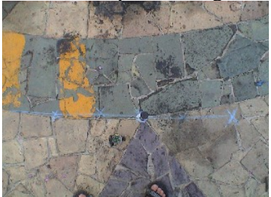
Another photo of the shadow path, taken from directly the top of the stick.
